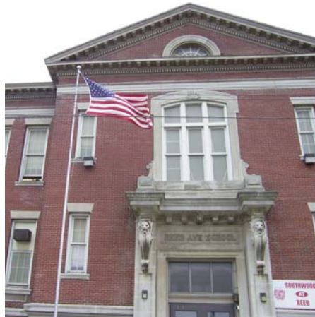
REEB ELEMENTARY SCHOOL, COLUMBUS, OHIO
