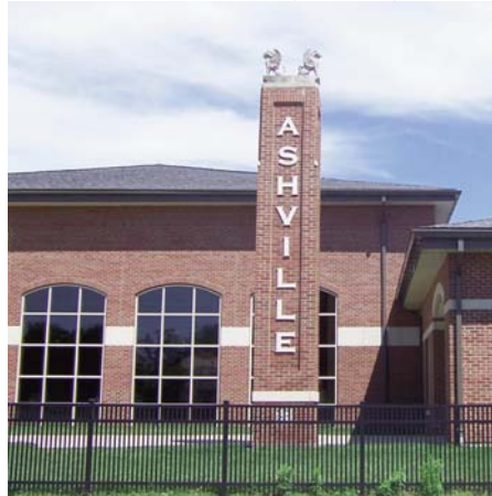
ASHVILLE ELEMENTARY SCHOOL, ASHVILLE, OHIO
