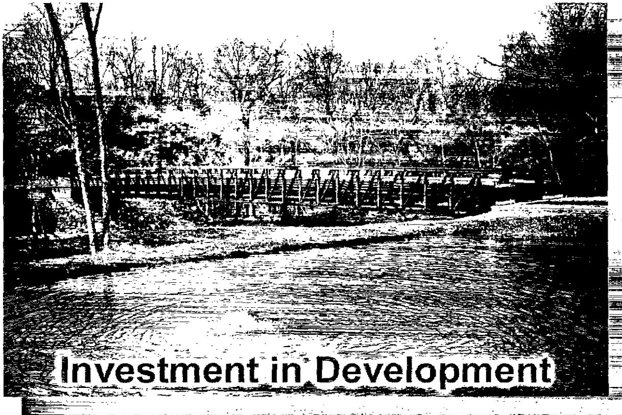
James Ranch Bridge connecting Creekside Trail to Fairground Recreation Center
