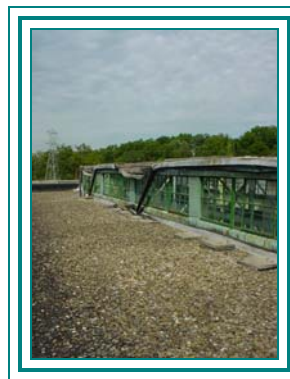
Condition of the roof prior to construction
