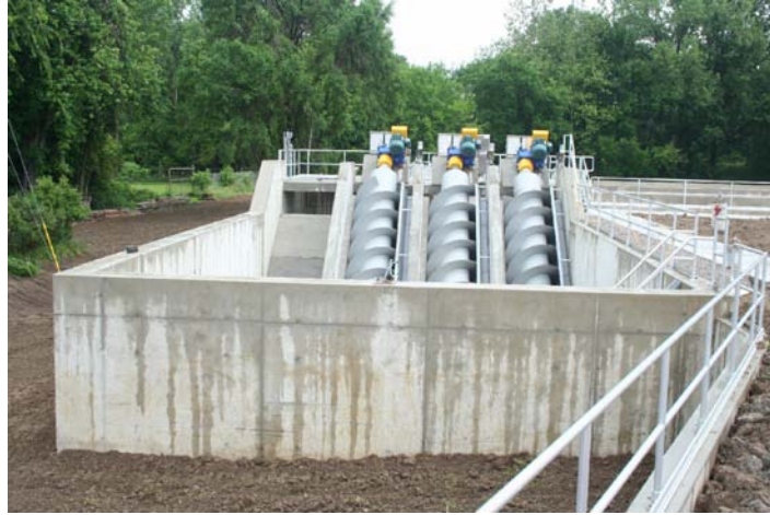
Raw Effluent Building
