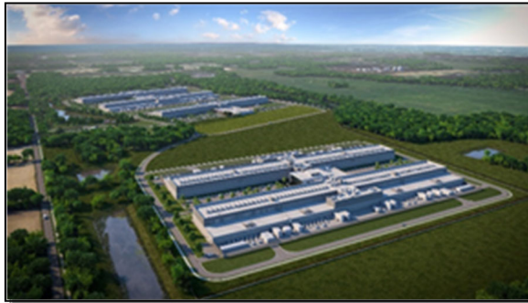
Figure 4 – Facebook New Albany Data Center
